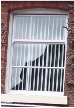
Photograph 12: 3 over 6 Timber Sash
