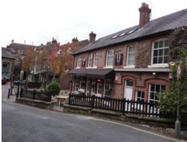
Photograph 33: Brick Wall with Stone Coping
