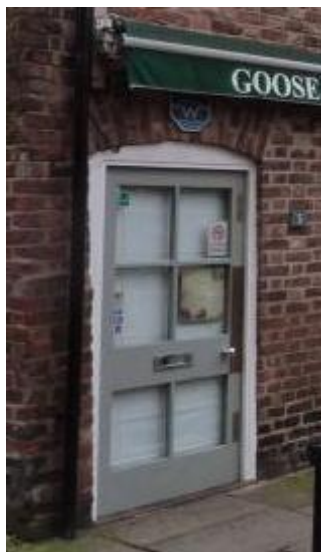
Photograph 21: Door with Soldier Arch
