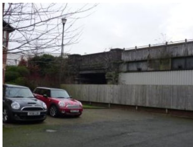
Photograph 34: Former Railway Bridge
