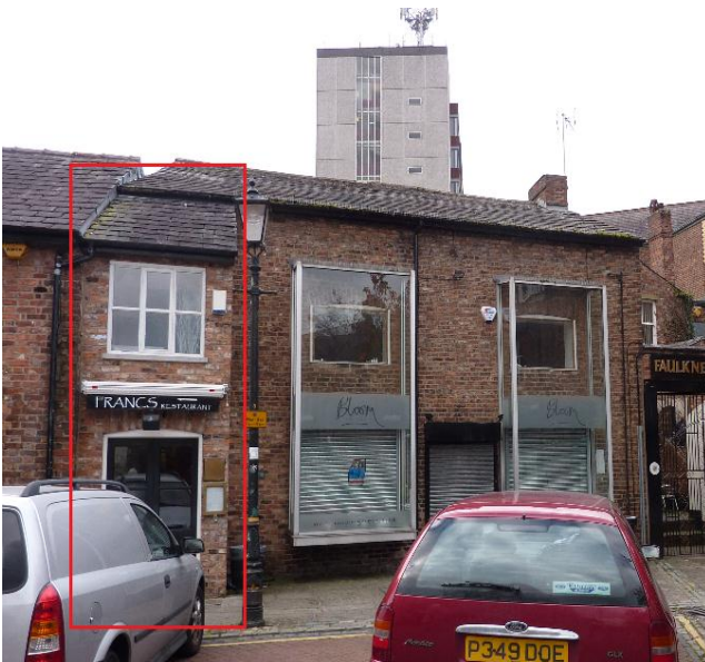
Photograph 27: Areas of Recent Alteration Extension
