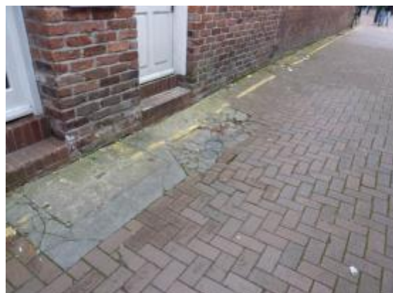
Photograph 45: Back Grafton Street
